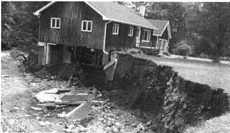
The photo on the left is an example of the extent of fluvial erosion which occurred during Tropical Storm Irene resulting in extensive loss of property and home damage in Windsor County
