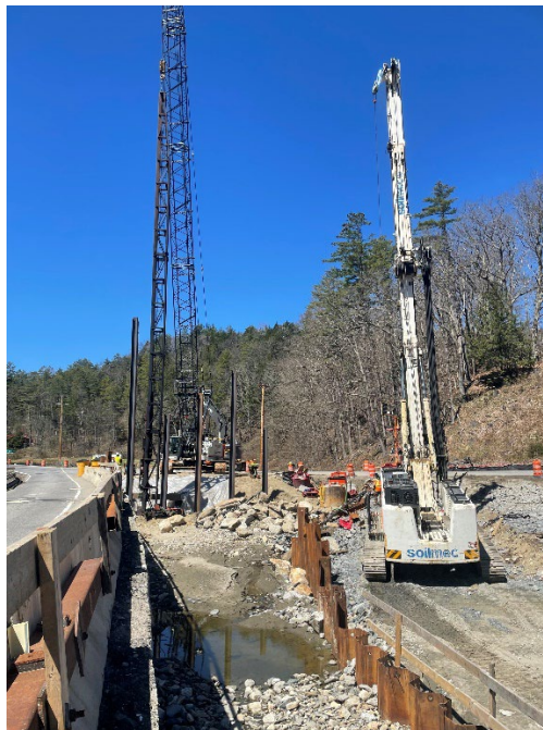
Crews install the pile foundation at the first bridge abutment.
