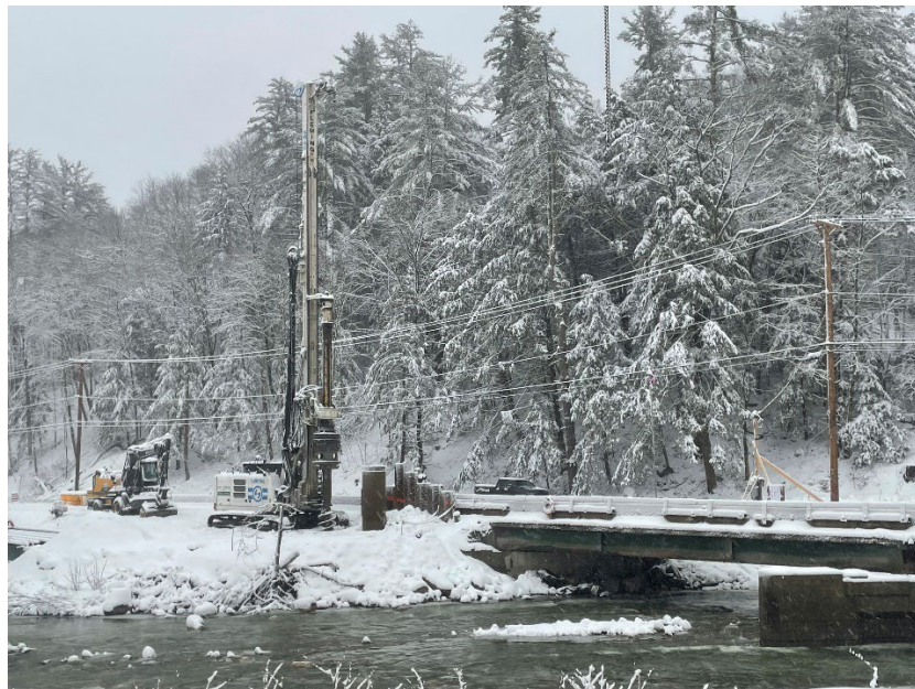
Crews pre-drill for the pile foundations at the second bridge abutment.
